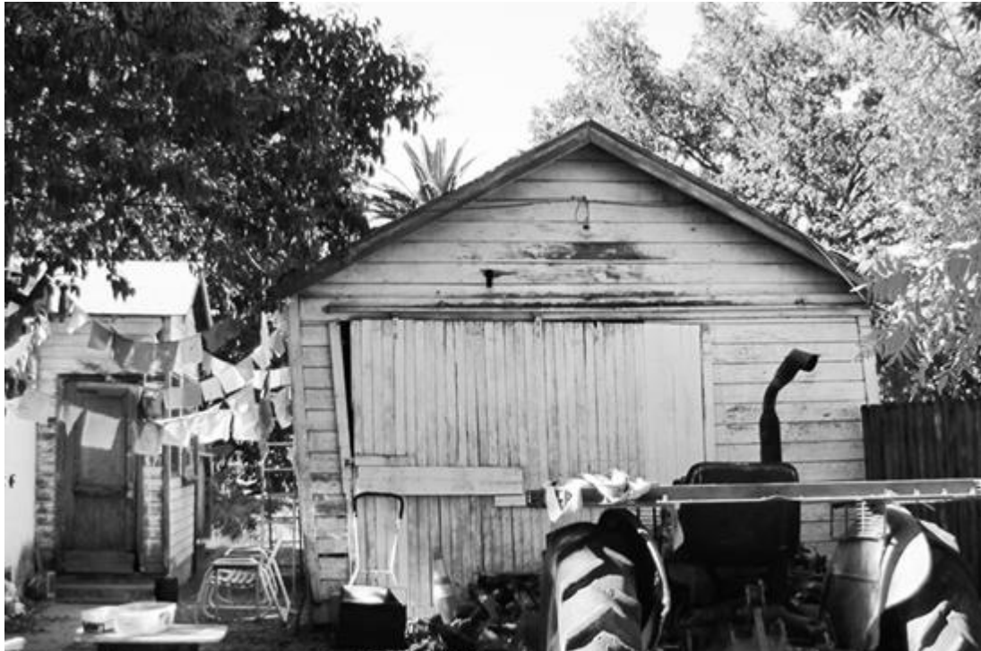
Photo A. South elevation of garage, 115 Hickory Lane. Note leaning wall at left.
