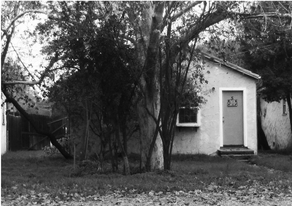
Photo S-12. 1233 Olive Drive, Unit 5, west elevation.
