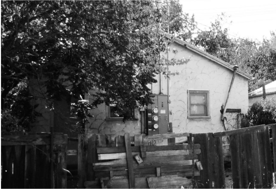
Photo S-13. 1233 Olive Drive, Unit 5, east elevation.
