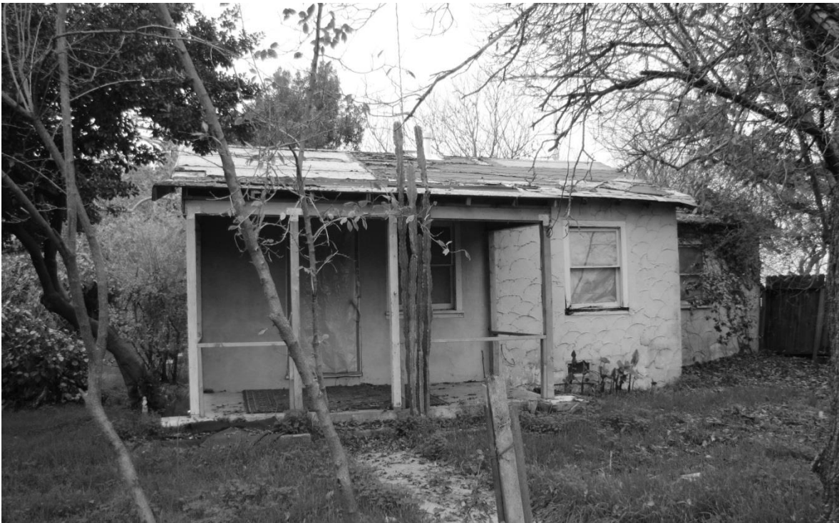
Photo S-8. 1233 Olive Drive, Unit 4, south elevation.
