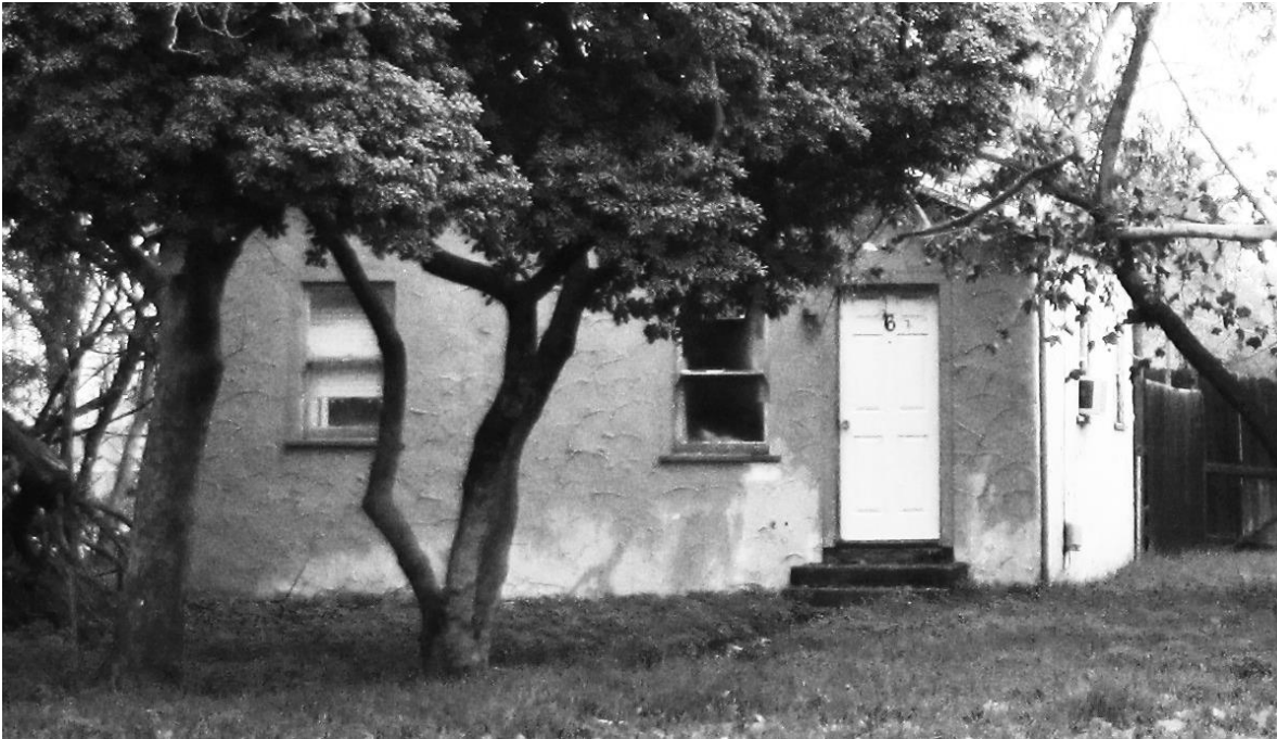
Photo I. West elevation of Unit 6. Stucco has been added over the original wood siding.
