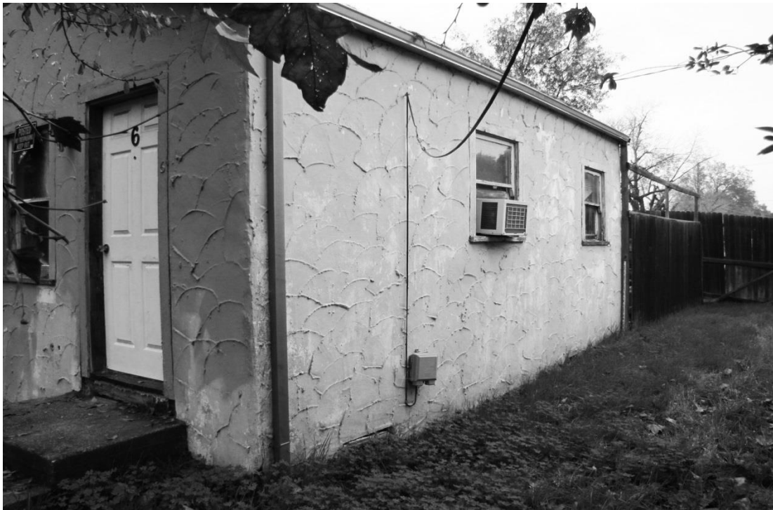
Photo S-14. 1233 Olive Drive, Unit 6, south elevation.
