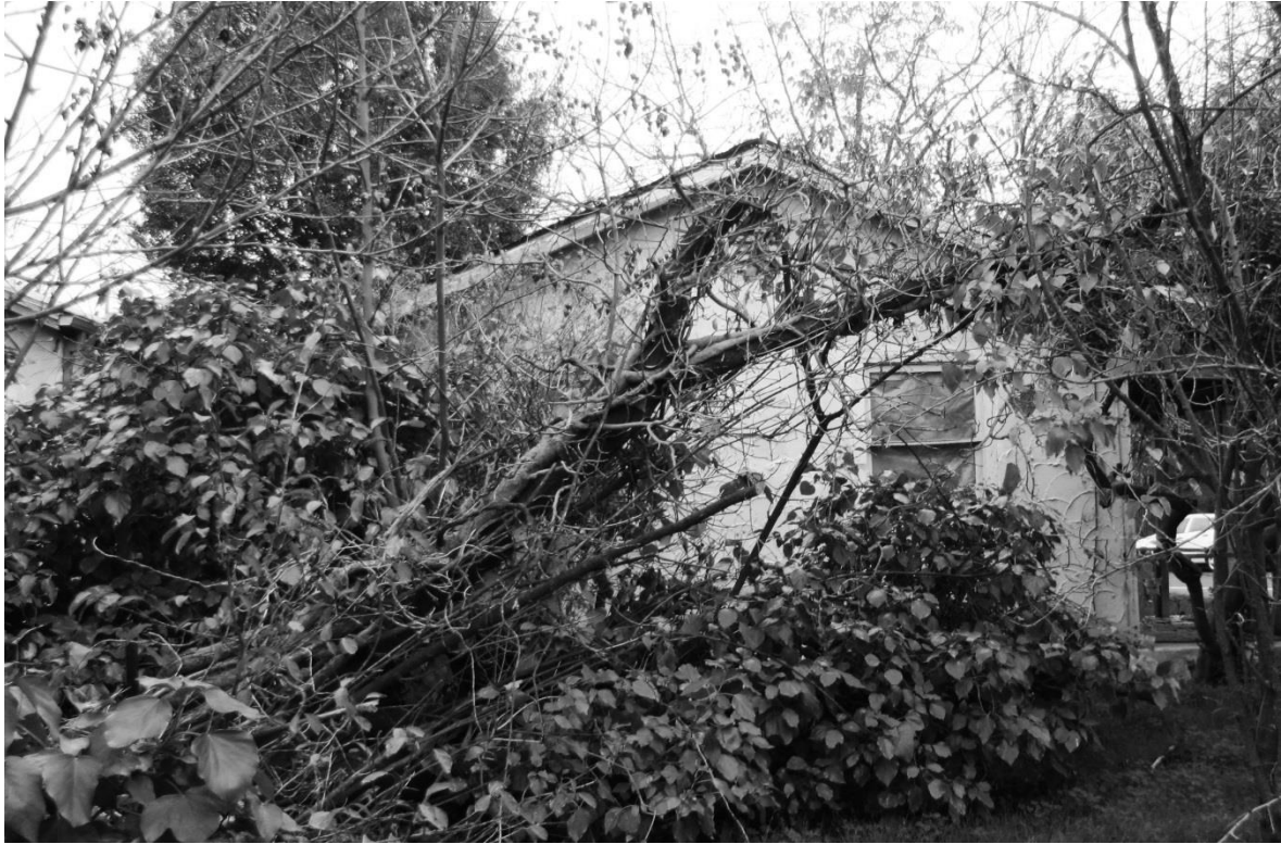
Photo S-9. 1233 Olive Drive, Unit 4, south elevation.
