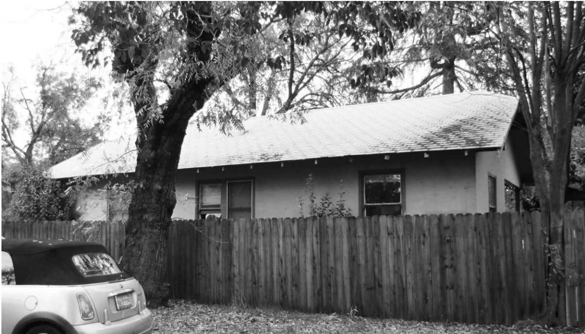
Photo S-3. Residence, 115 Hickory Lane, west elevation.
