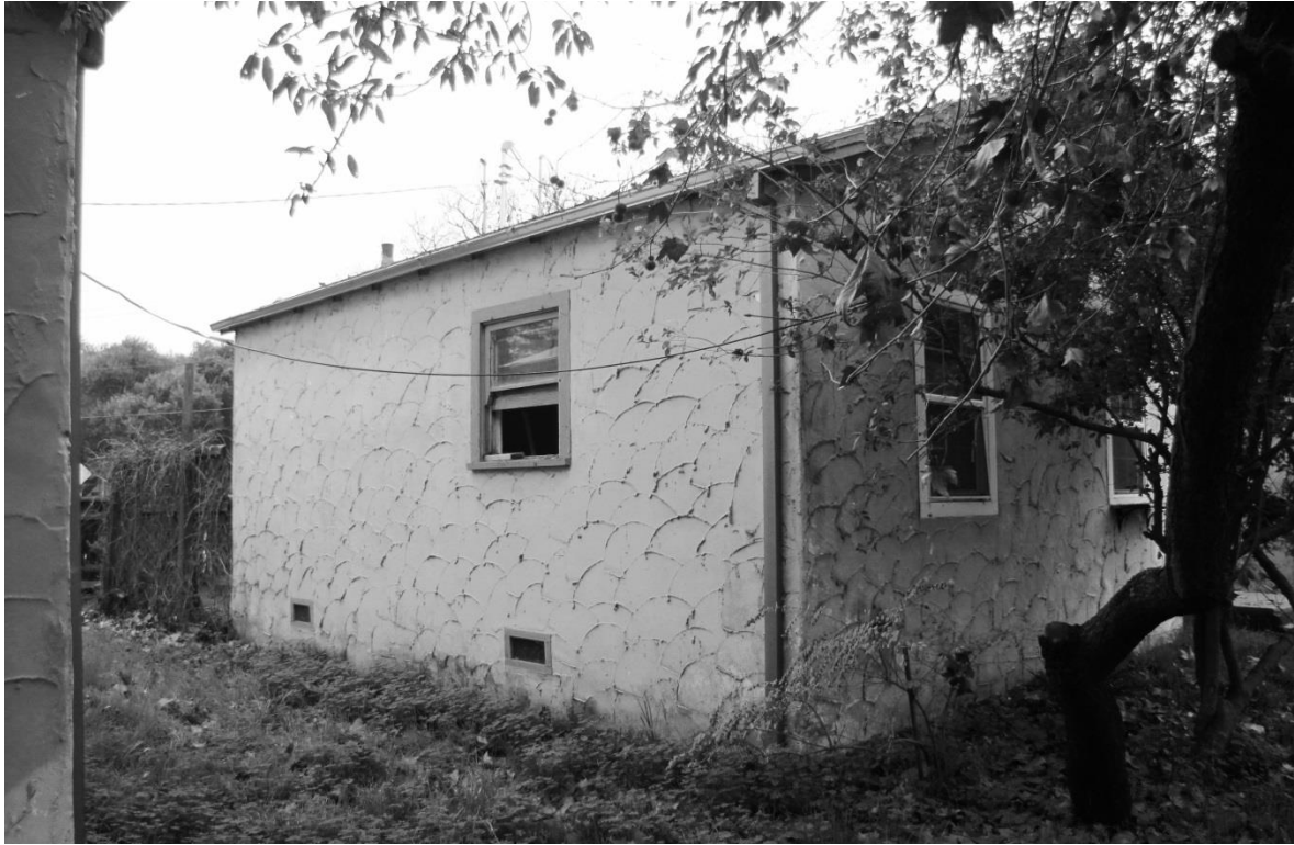
Photo S-11. 1233 Olive Drive, Unit 5, north elevation.
