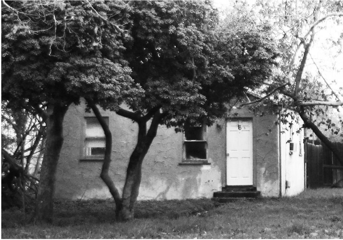
Photo S-15. 1233 Olive Drive, Unit 6, west elevation.
