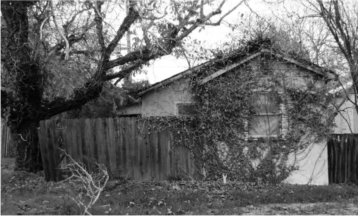
Photo S-7. 1233 Olive Drive, Unit 4, east elevation.
