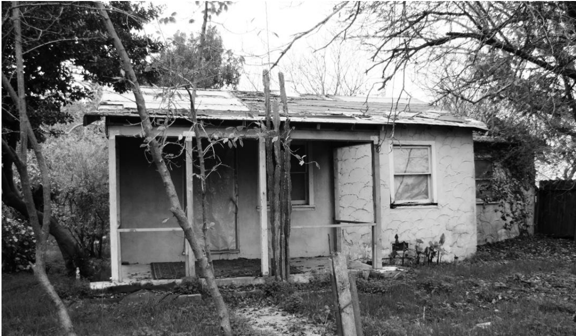
Photo G. South elevation of Unit 4, with entrance and porch facing Olive Drive. Roof is in poor condition. The porch has been identified as a safety hazard.
