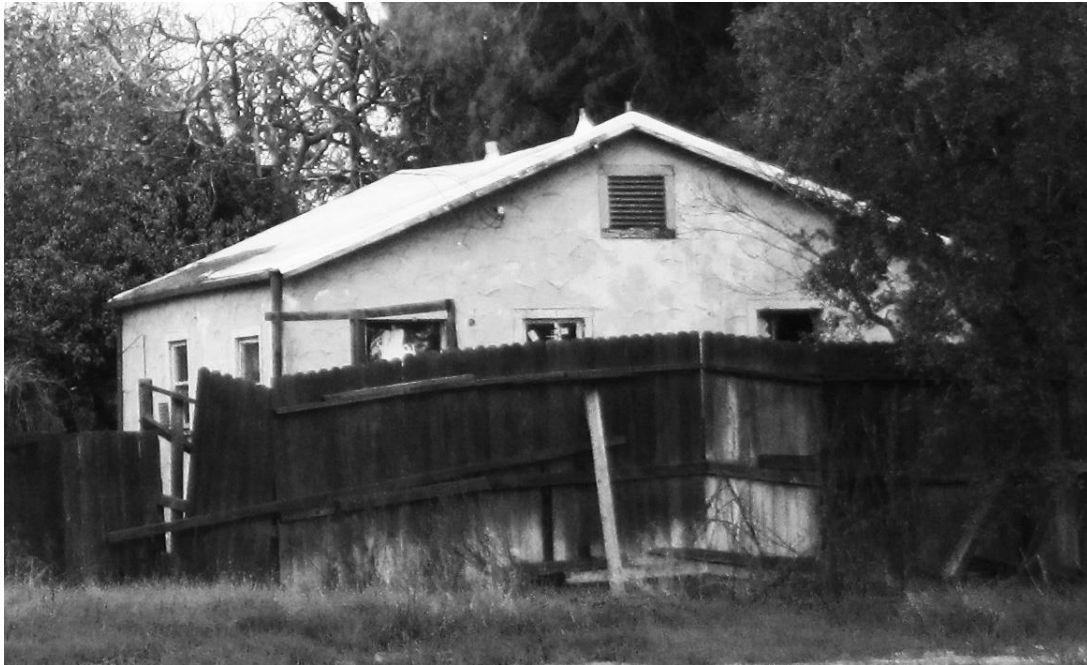
Photo S-16. 1233 Olive Drive, Unit 6, east elevation.
