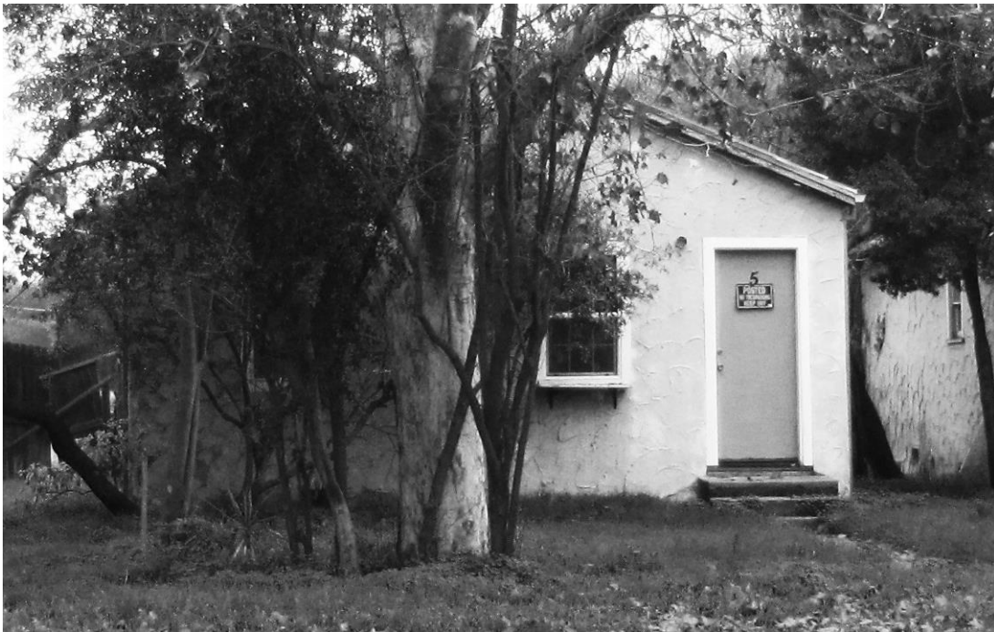
Photo H. West elevation of Unit 5. Original windows and the entrance door have been replaced, with stucco added over the original wood siding.
