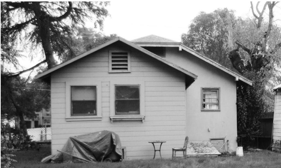
Photo S-4. Residence, 115 Hickory Lane, north elevation.
