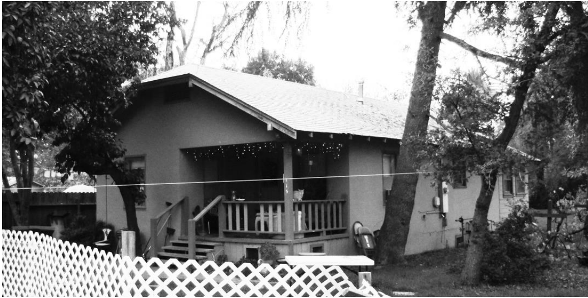
Photo C. Porch on southeast corner of residence, 115 Hickory Lane.
